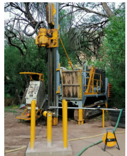
Well installation at the Sonora Lithium Project Bacanora Minerals
